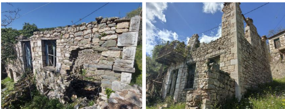
Image 3-30. Cornerstones with roughly carved faces with a carved decorative strip around their perimeter (left), cornerstones with careful carving over the entire surface of their faces (right). In the upper part of the corner there is a decorative motif on a cornerstone as well as the date of construction of the building. Source: NTUA Research Team, 2023.
