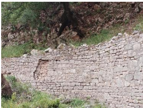
Image 3-59. Damage to the stone-built retaining wall of the path leading up to the bridge from the east. Source: NTUA Research Team, 2023.
