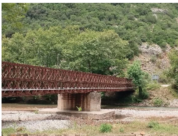
Image 3-60. The Bailey bridge has reinforced concrete piers. Basic maintenance of its metal elements is required. Source: NTUA Research Team, 2023.
