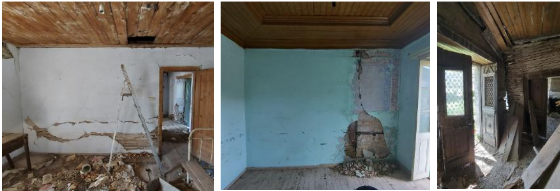
Figure 3-34. Wooden partition walls made of bagdati on the first floor (left-House "of the Teacher" and center-House "of Swolos") and on the ground floor (right-House of Nikopoulos). Source: NTUA Research Team, 2023.
