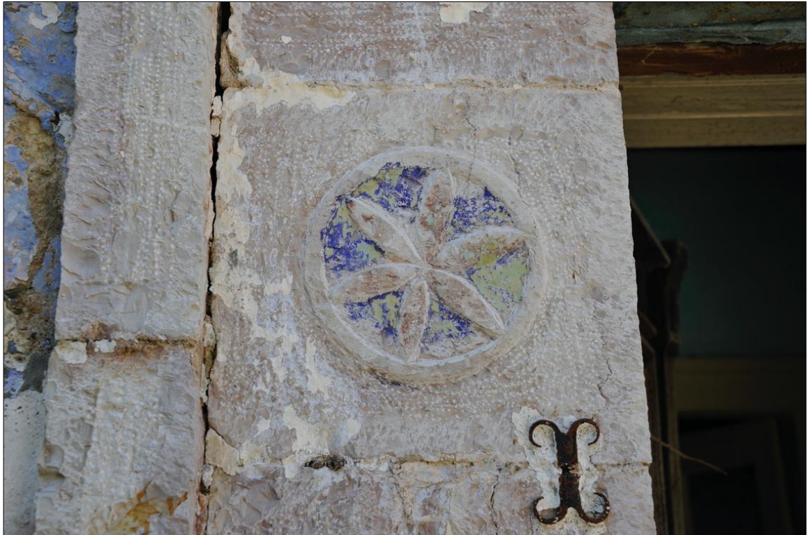
Image 3-11. Decorative relief; rosette on a doorpost block and hammered metal "fork" connector, anchoring the wooden frame. Source: NTUA Research Team, 2023.
