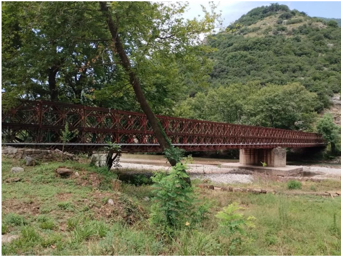
Image 2-23. The new Bailey-type metal bridge over the Megdova. It was built by the army in 1947. At a distance of about 50 meters downstream, the "kareli" - the aerial transport cage - crossed the river. Source: NTUA Research Team, 2023.
