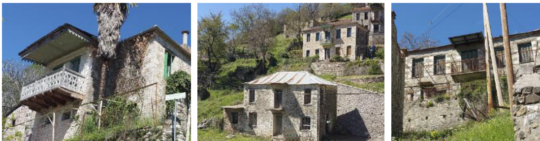
Image 3-44. The best preserved wooden balcony of the House of "Svólos" (left). Balconies made of reinforced concrete that replaced wooden ones. Source: NTUA Research Team, 2023.
