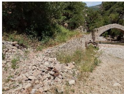
Image 3-59. Damage to the stone-built retaining wall of the path leading up to the bridge from the east. Source: NTUA Research Team, 2023.
