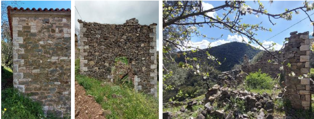
Image 3-31. Argolithodomies with gray stones and white cornerstones. (area of the "Teacher's" House). Source: NTUA Research Team, 2023.
