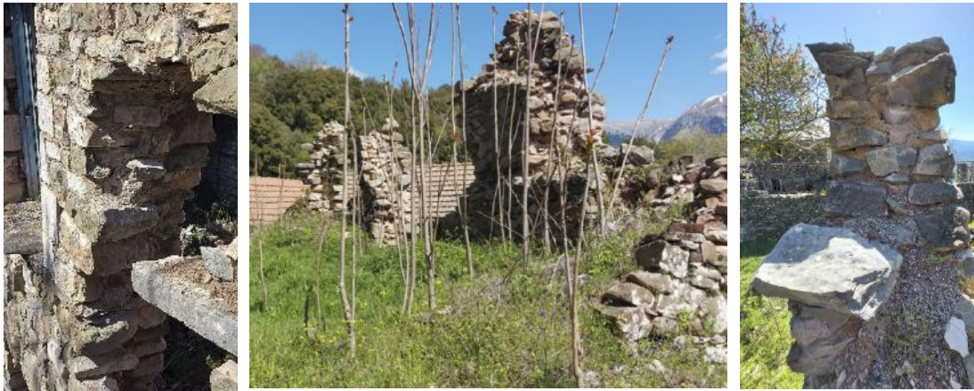
Image 3-29. Three-layer masonry. Source: NTUA Research Team, 2023.
